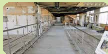
➡The walls and ceiling are stripped off on the first floor
